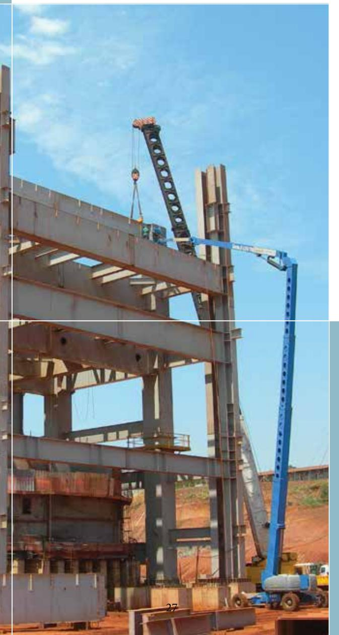
*Votorantim Metals has contracted Brafer to manufacture and erect 3,700 tons of structures for the Steel Processing Plant of Iron-Nickel, located in Niquelândia- GO. The structures are present in the secondary crushing plant, loading and unloading of the calcination furnace and Pyrometallurgy. For the Pyrometallurgy Plant, Brafer fabricated 44 ton box-columns, this being the largest piece ever made in the company history.*
