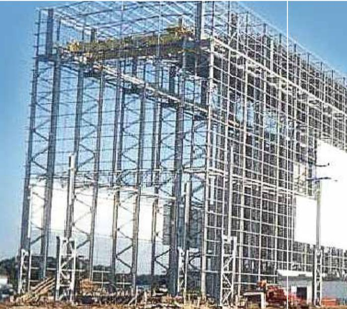
*Cold rolling Complex, located in Araucária, Paraná. The galvanizing building is 50 meters high, and spans 25 meters. The total weight supplied is 3,400 tons.*
