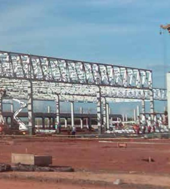
*Hired by the South Korean company Hyundai Motors, Brafer was responsible for the manufacturing and erecting of the metal roof of a building that make up the automaker's new plant in Piracicaba-SP. Providing more than 2.000 tons of structures with an internationally recognized level of quality, Brafer served an extremely short production and erection schedule, making use of the company's two plants, happening completely synchronized.*
